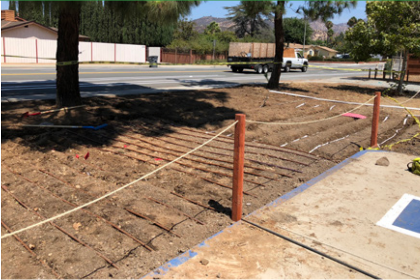
Irrigation install complete. Standard drip installed in foreground, RDI is installed background.
